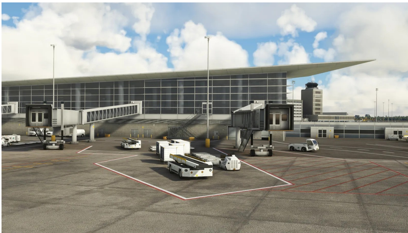
Ground support equipment staged at the Winnipeg terminal
