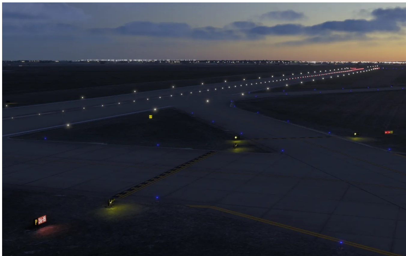
Taxiway and runway lighting at dusk
