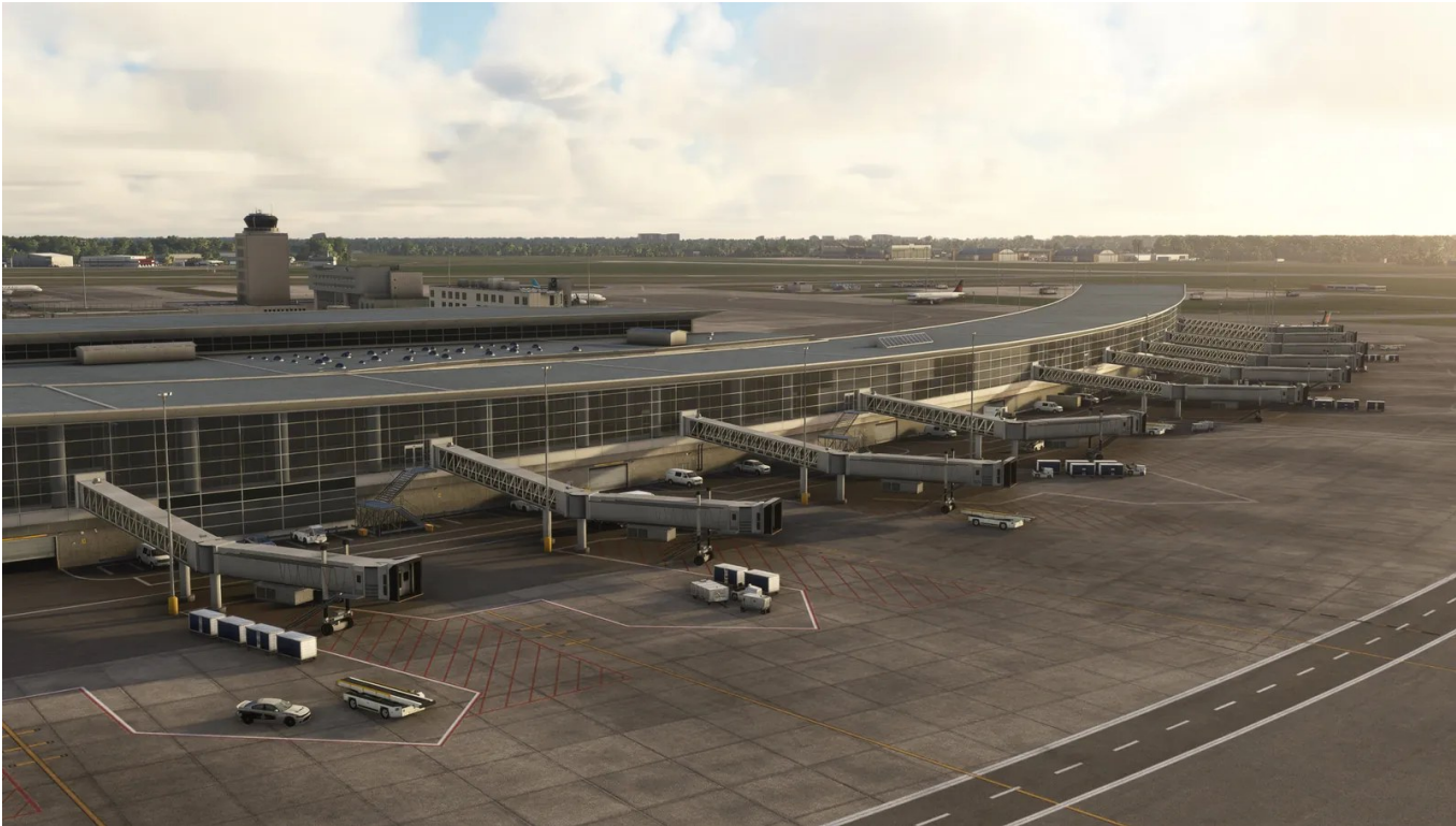
Terminal gates and boarding bridges.
